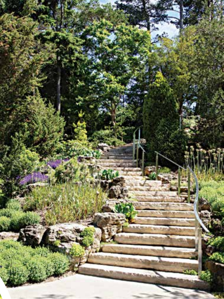
▲ This old stairway has been retained in the redesign but the new handrail increases safety. This view was used for the cover photo of Escarpment Views , Spring 2010.
